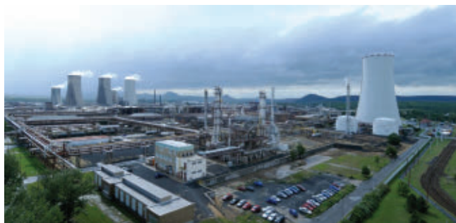
Unipetrol AS has rebuilt a steam cracker at its Chempark Zaluži facility at Litvinov, Czech Republic. Photo from Unipetrol.
